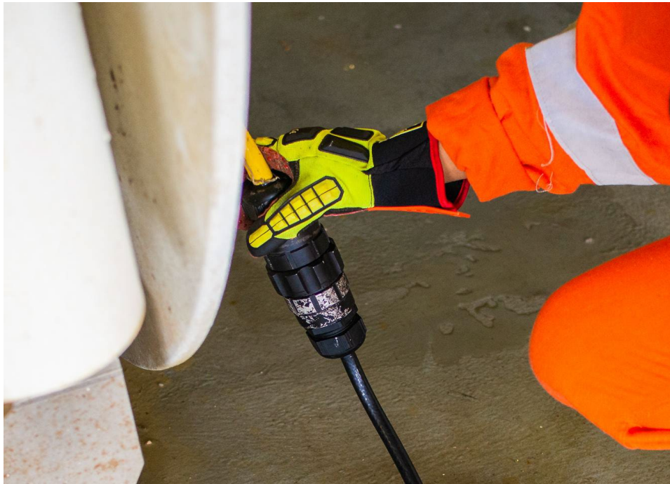
Figure 5. Connection between tow cable and deck cable located on winch.
