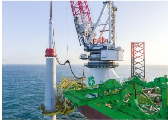
Pile Driving of a Monopile
