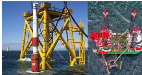
Pile Driving of a Jacket Pile
