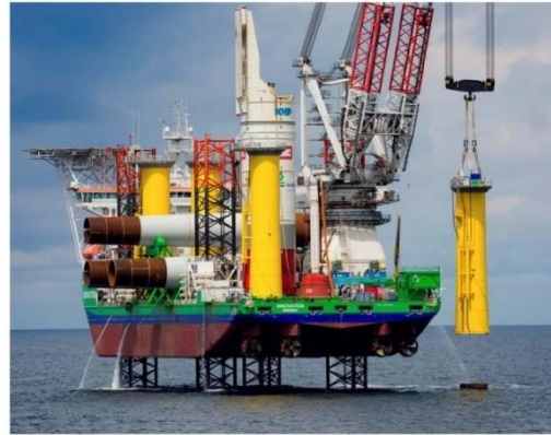
Transition Piece Installation from a Jack-Up Vessel
