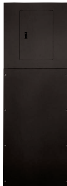
Panel Skirt Completely Installed
