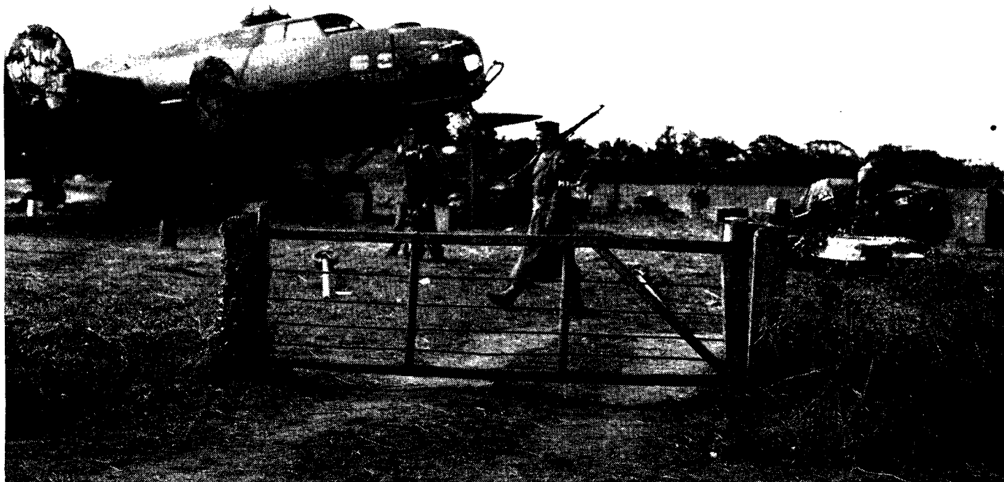
Mobile repair units for crashed aircraft, like medical units for injured personnel, follow their planes and make emergency repairs. The 8th Air Service Command maintains units which travel wherever disabled planes have landed. This plane's four engines and ball-turret were damaged in an emergency landing, but the bomber was able to take off from a make-shift runway after the mobile unit had completed the repair job.
