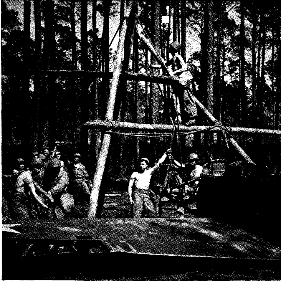
At Mississippi's "Guadalcanal" all devices are strictly homemade. Students at left bring up a log shoring frame as a wing rest once the fuselage is hoisted sufficiently.
