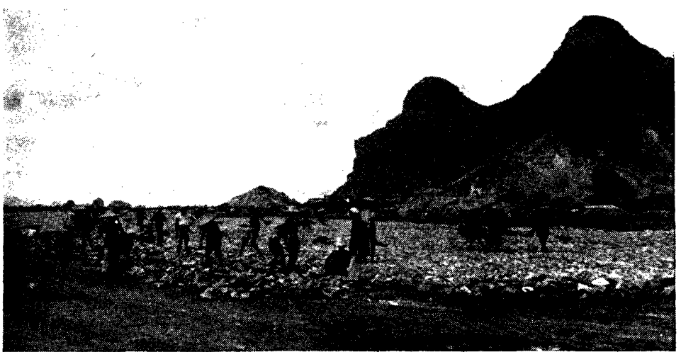
Although the Chinese have to quarry, crush, transport and lay the rock by hand, they succeed in constructing excellent runways of stone, two feet thick. The bed is cemented with a paste of mud.
