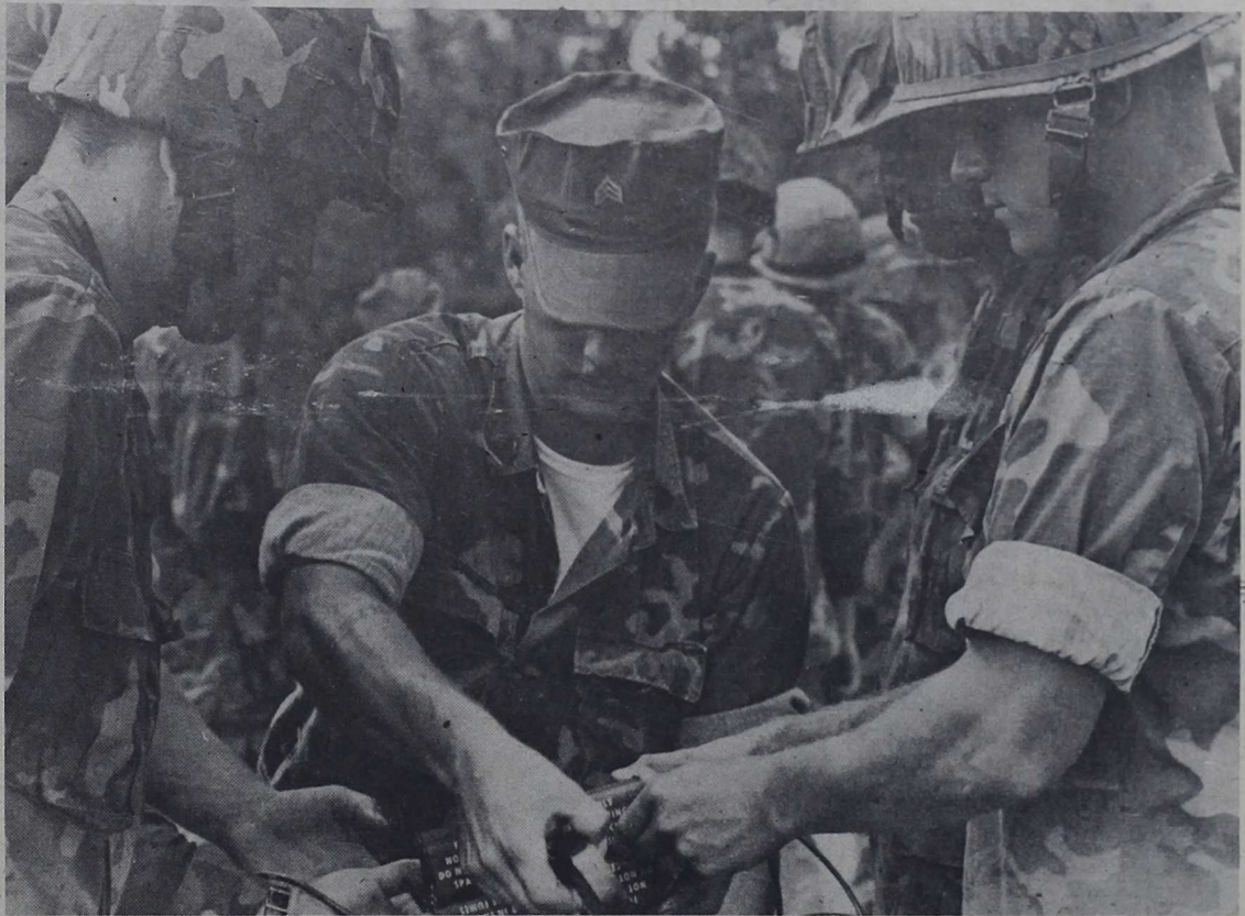
FINAL TOUCH — Strapping four blocks of TNT together with black electric tape, Sgt. David H. Winger, 2nd Combat Engineer Battalion instructor, shows Marines from Battery D, 2/10, one method of surface detonation during a demolition class.
