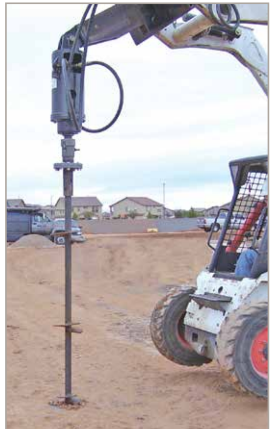
Typical MB Brace Badger Installation
