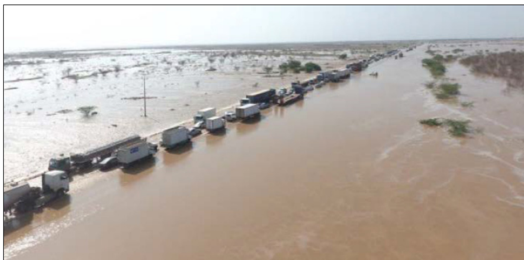
Figure 2. International Jizan–Jeddah road under the flooding of the Wadi Al-Lith [29].
