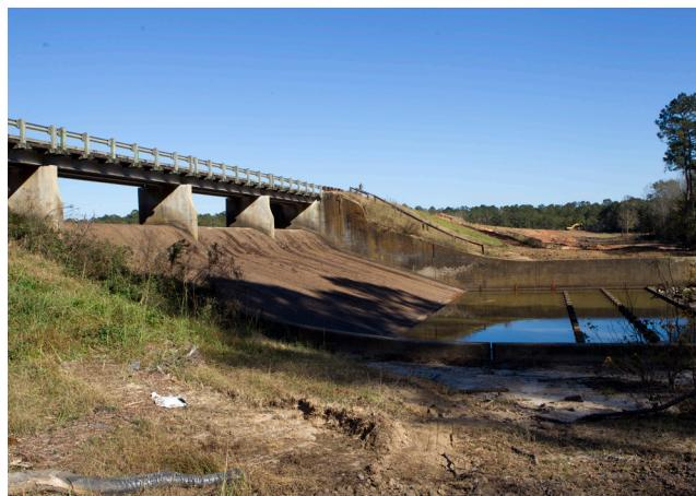
MDOT's employees did not hesitate to meet the challenge. MDOT crews worked around the clock to construct a channel to relieve pressure on the dam. The channel was approximately 600 feet long, 100 feet wide at the bottom, 200 feet wide at the top, and approximately 40 feet deep in certain places. It is estimated that there
