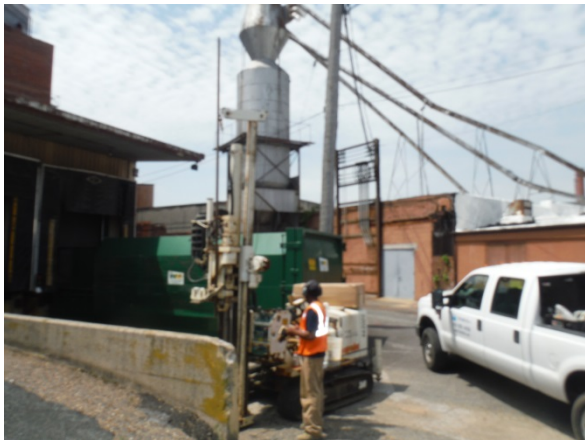
Photograph 9. Soil boring SB-6 location.
