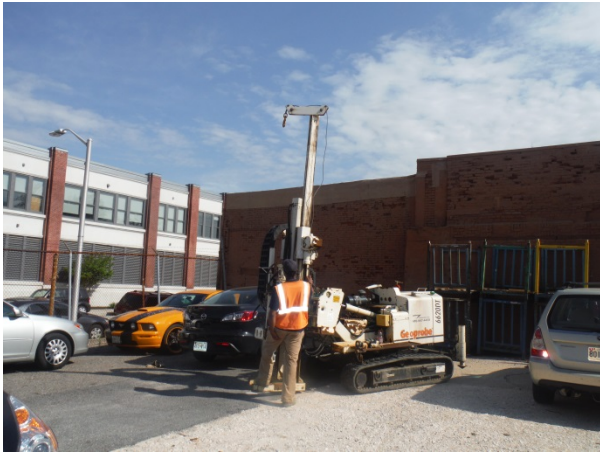
Photograph 11. Soil boring SB-7 location.
