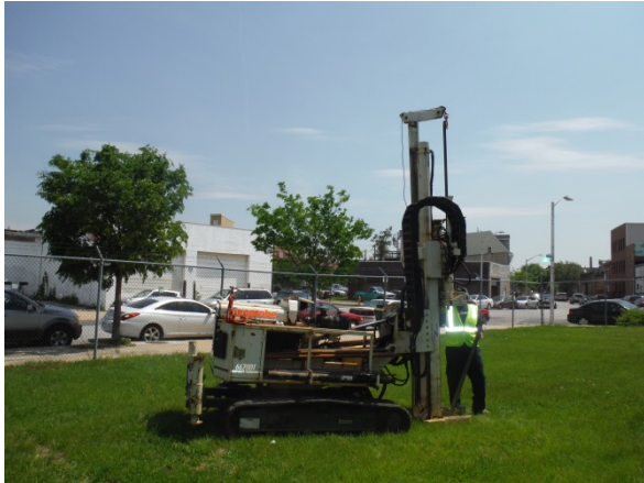
Photograph 9. Soil boring SB-5 location.
