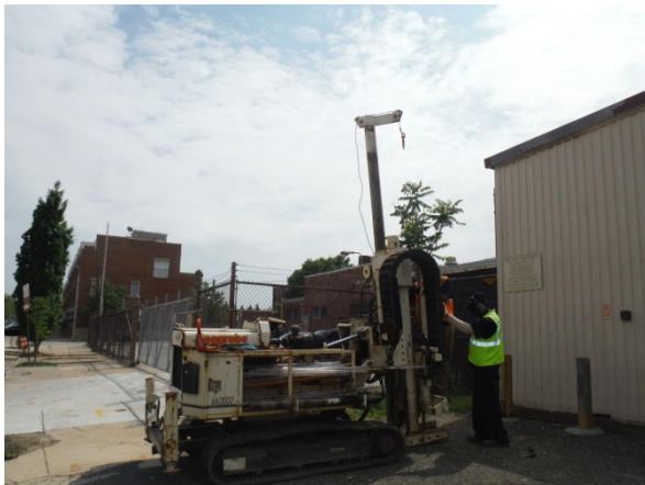
Photograph 3. Soil boring SB-2a location.
