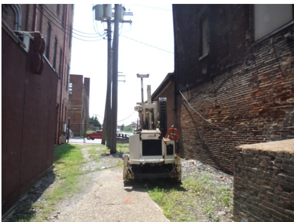
Photograph 15. Soil boring SB-10 location.
