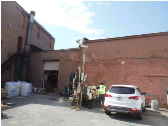
Photograph 5. Soil boring SB-3 location.
