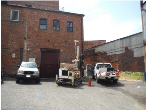
Photograph 7. Soil boring SB-4 location.
