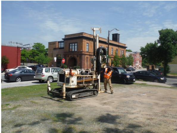
Photograph 1. Soil boring SB-1 location.
