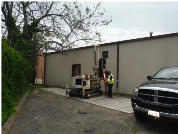
Photograph 19. Soil boring SB-12 location.
