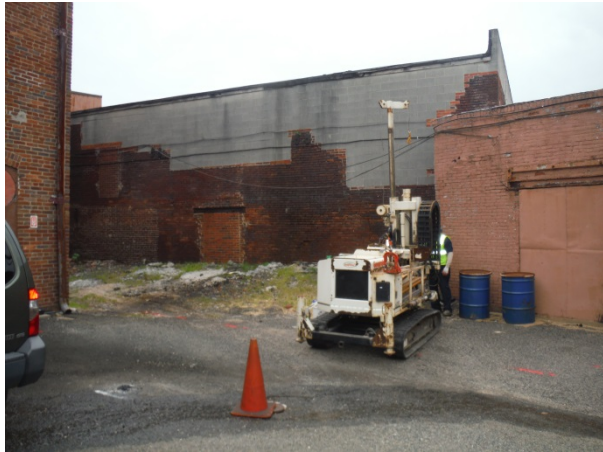
Photograph 17. Soil boring SB-11 location.
