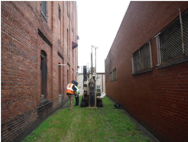
Photograph 13. Soil boring SB-9 location.
