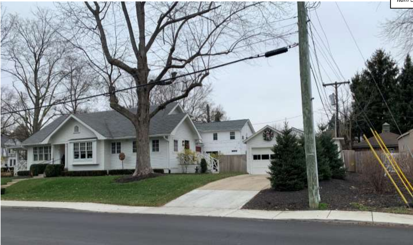
Photo of the single-family dwelling west of the site.
