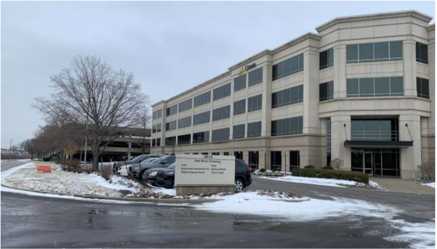
North façade of the subject property at 3815 River Crossing Parkway.
