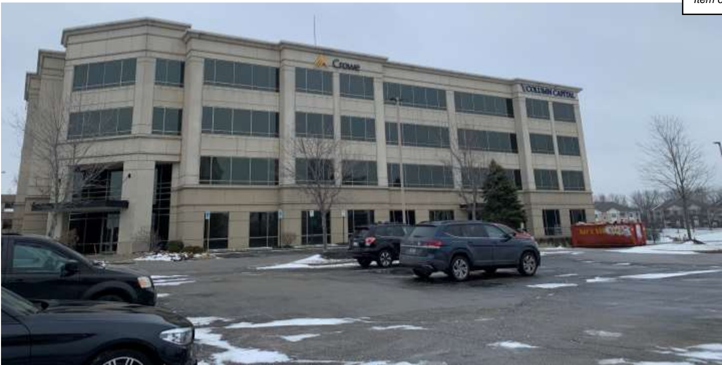
West façade of the subject property at 3815 River Crossing Parkway.
