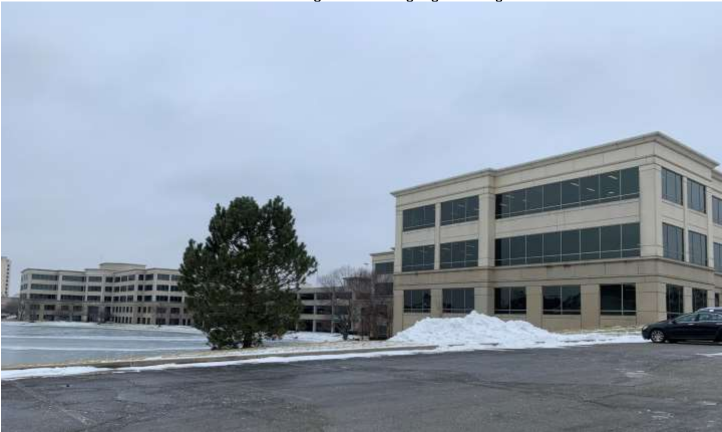
Photo of the south building facades.
