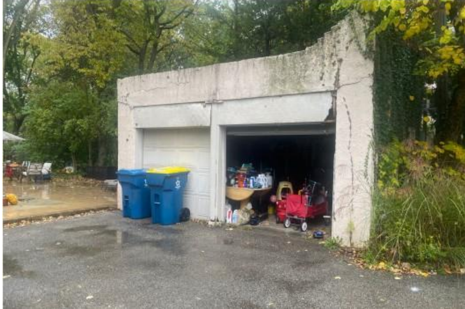
Photo 3: Southern Elevation of Existing Garage (taken October 2023)
