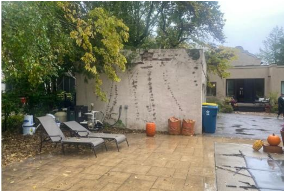
Photo 4: Western Elevation of Existing Garage (taken October 2023)
