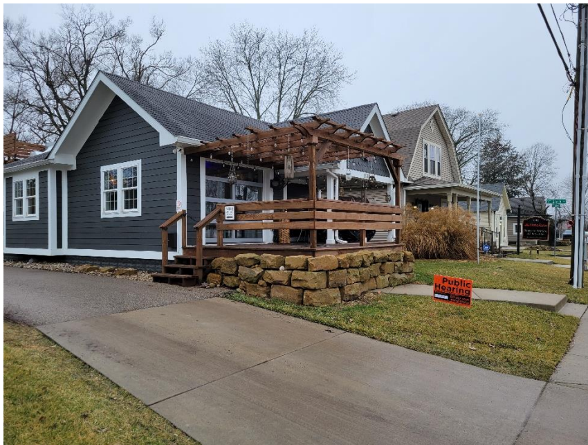
Photo 2: Covered Sidewalk Café Within ROW Viewed from Southeast
