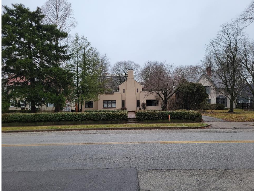
Photo 1: Existing Residence Viewed from Across Pennsylvania (East)
