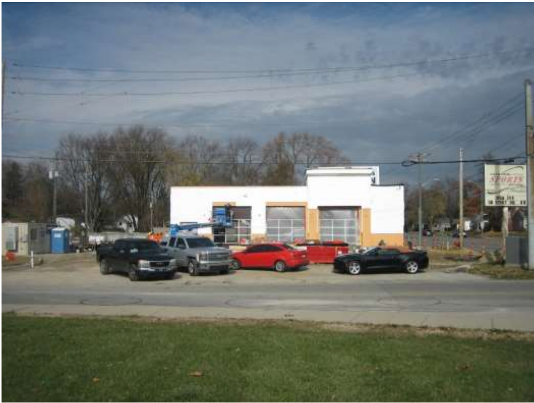
View of subject site, proposed building under construction, looking north from East 56 th Street.
