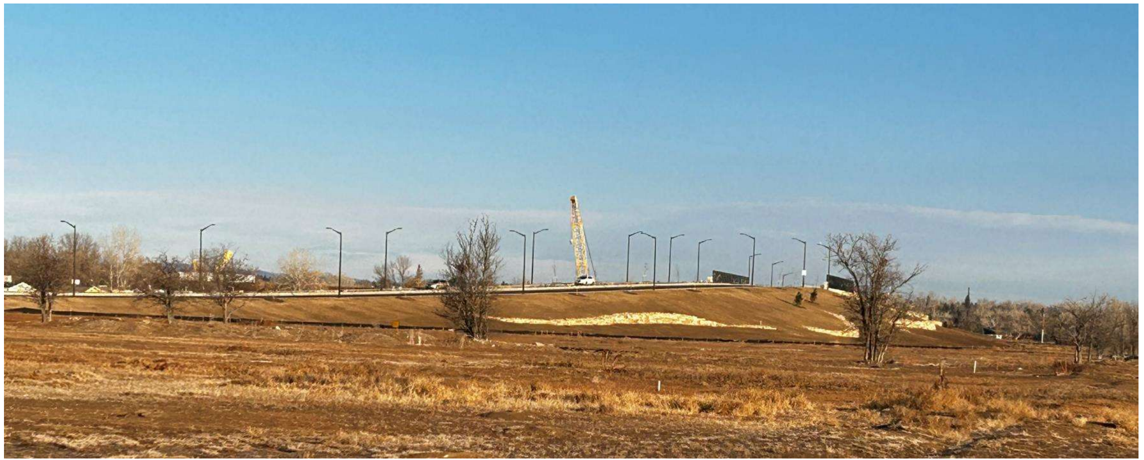
View from site looking north/northwest at Lemay Avenue overpass over Vine Drive
