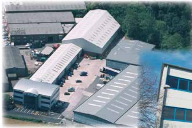
Cembre Ltd. factory in Curdworth (Birmingham)
