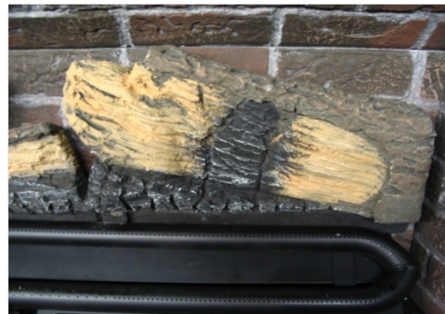
Log "B" installed correctly
