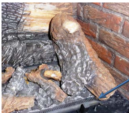
Log "H" front tip sits on flat crimp of front burner
