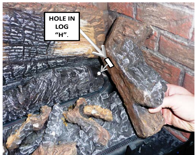
Log "H" front tip sits on flat crimp of front burner
