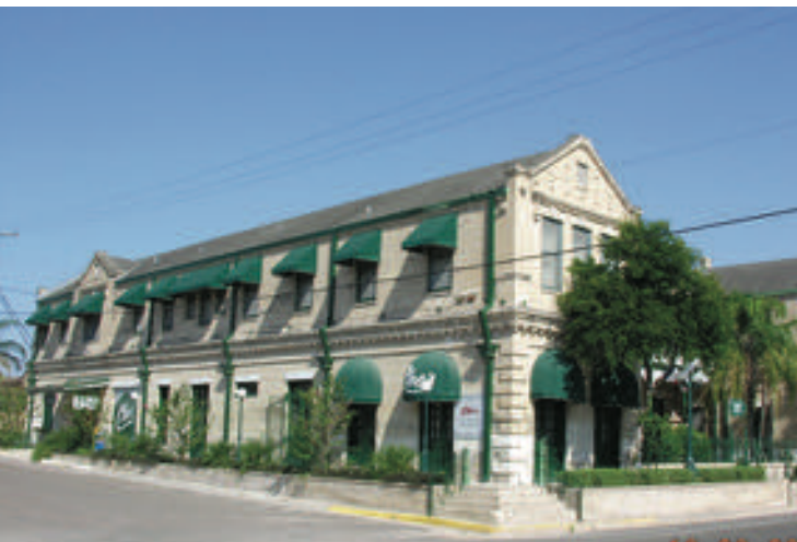
(top) In Río Grande City, a recently rehabilitated courtyard interconnects a complex of historic residences. The stone wall separating the patio from the street is a composite of lime mortar and stone, known as cal y canto and commonly used in the mid-1800s along the lower border region. (above) The patio-centered La Borde House, built in the 1890s and 1910s, was recently restored.
