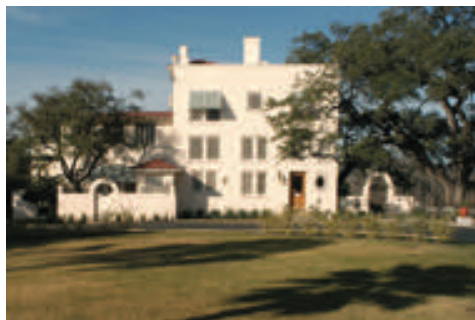
Laguna Gloria-Driscoll Villa Restoration
