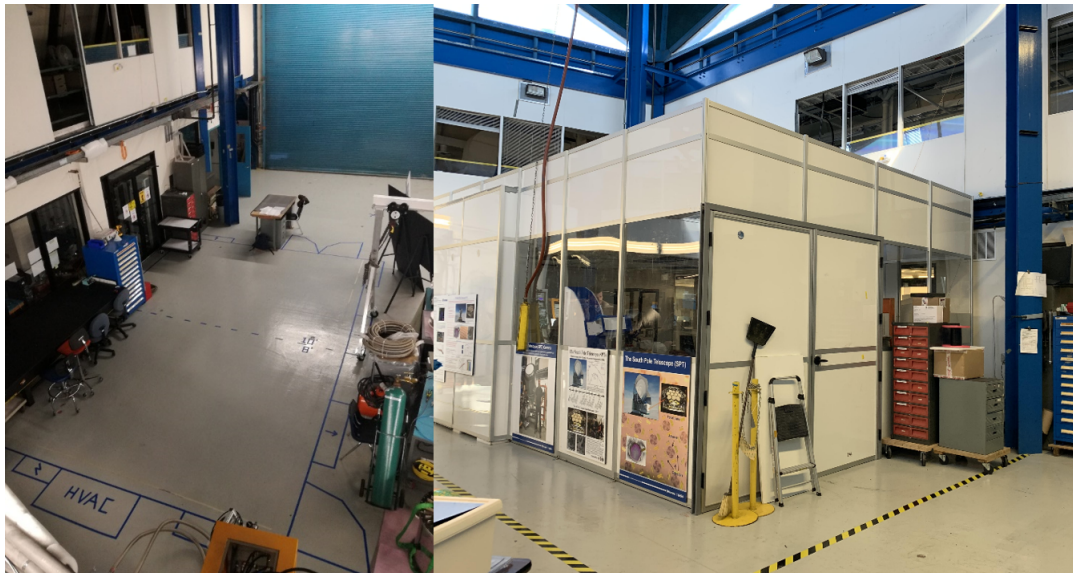
Figure 26: A picture of the cleanroom layout taped on the floor before the installation (left). A picture of the actual cleanroom installed at SiDet (right).
