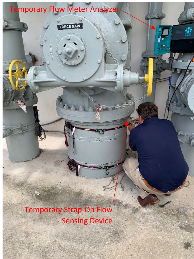
Installation of Temporary Flow Metering Device
