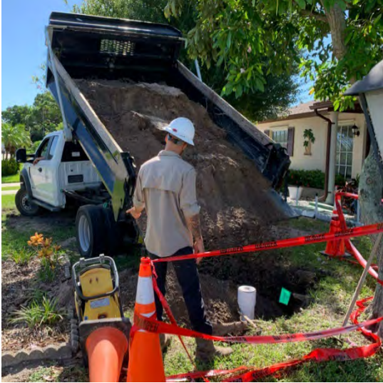
Pictured at left: Alex Smith is directing Tommy Cox as he offloads fill dirt at a recently installed cleanout. At right: Tommy Cox, operates a compactor utilizing hearing protection, gloves, and safety boots.
