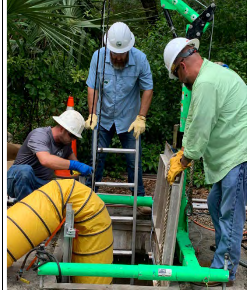
Pictured at left: Jason Broadrick enters LS 266 while Confined Space Writer John Voss (Construction Manager) supervises the entry and Attendant Ryan Chernekoff monitors activity. At Rt: Robbie Spires along with Ryan and John, support the rehab effort Jason is performing in the pit.
