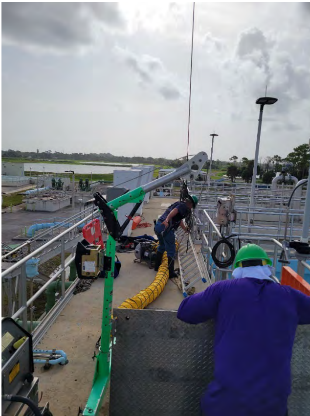
Filter Backwash Pump Removal and Maintenance
