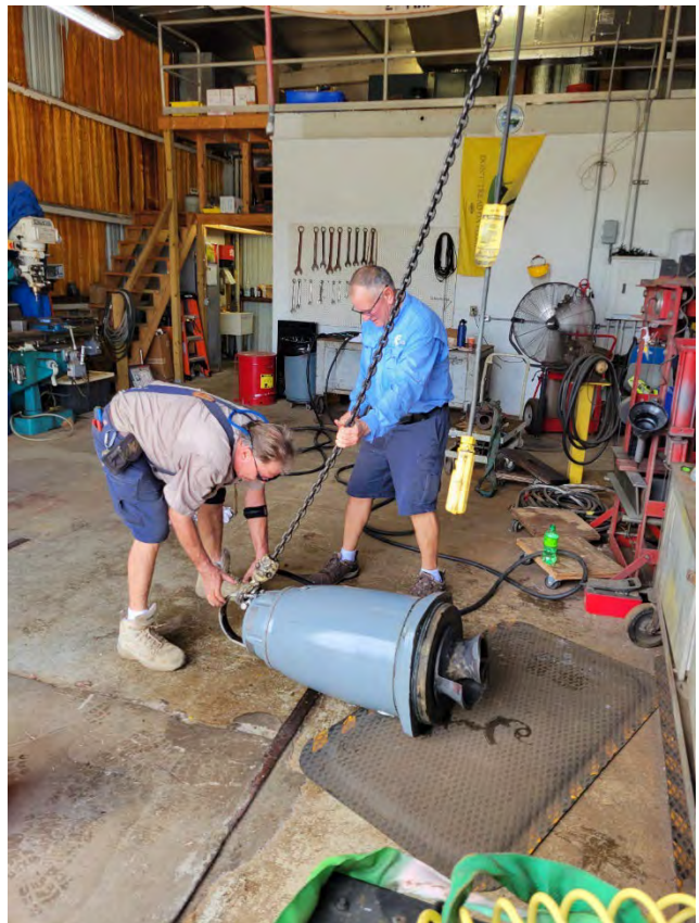
Filter Backwash Pump Removal and Maintenance
