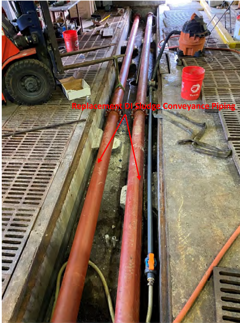
Replacement Sludge Conveyance Piping
