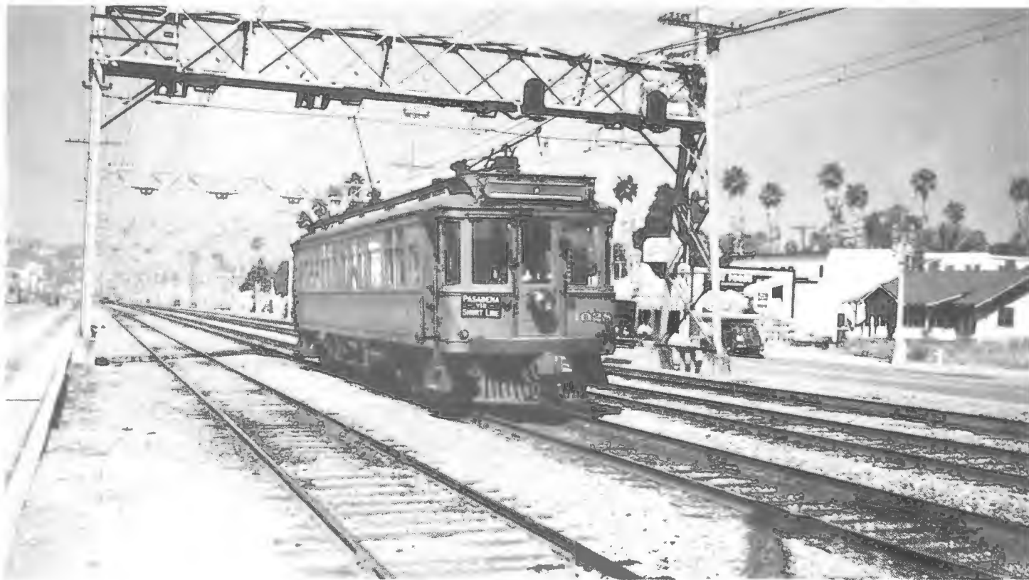
Below, car 1028 (famous old Orange Empire Trolley Trip car) speeds along the "dream" right of way through El Sereno en route to Pasadena via the Short Line; circa 1945. (AA-AH)
