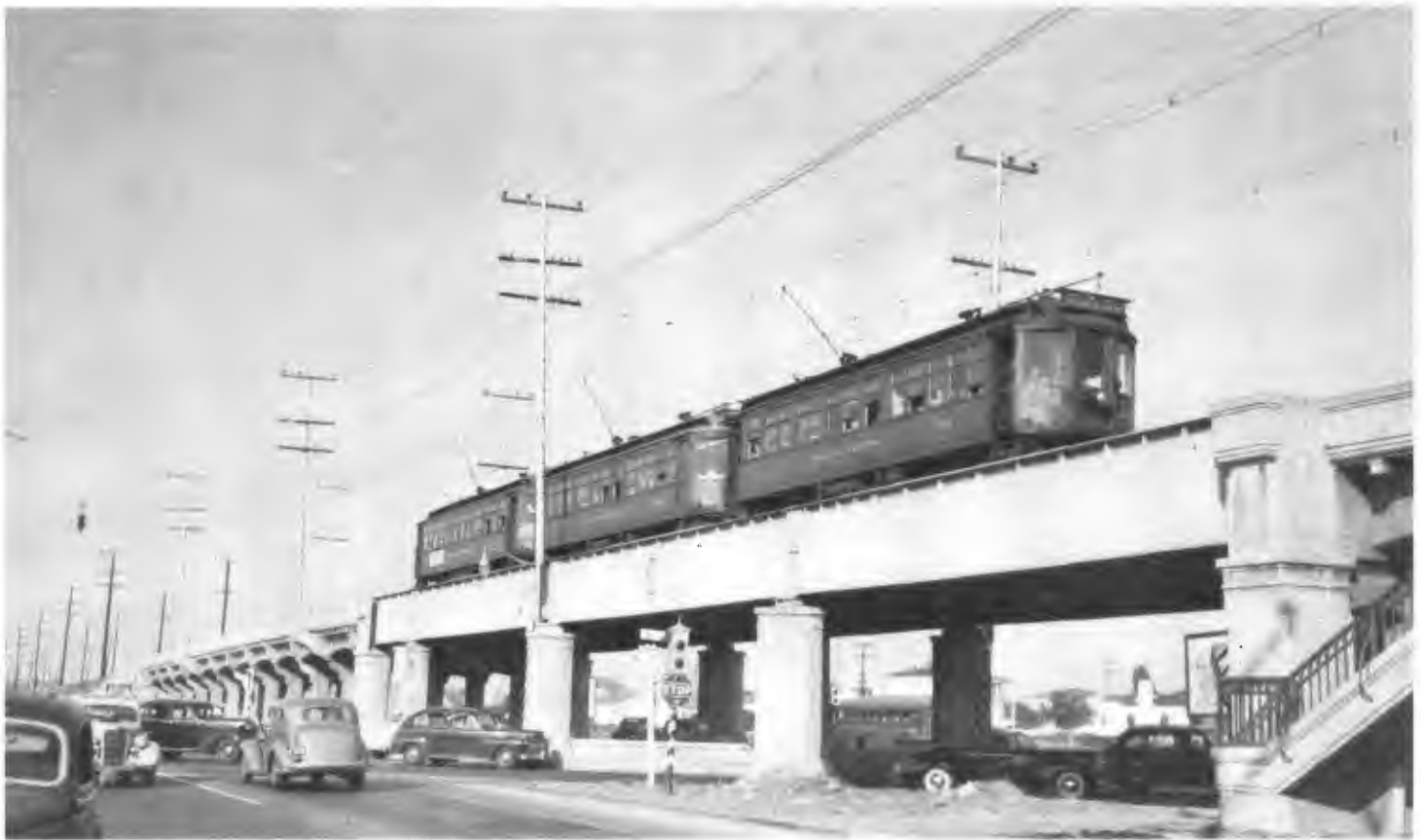
Three cars loaded down with holiday seekers speed over the massive La Cienega grade separation in 1937. Car 972 heads the impressive Venice Short Line train. (AA-AH)
