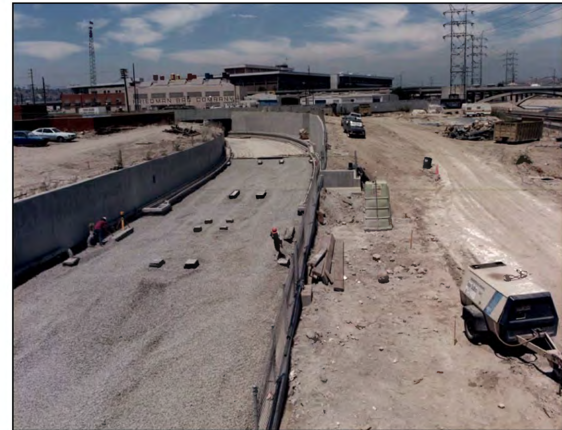
Photo No. 7. Sub-ballast placed on the base of slab in the "U" wall structure area, East Portal Entrance (south of LAUS). Looking north towards LAUS. Photo taken: 07/30/90. Source: SCRTD, 1990a.
