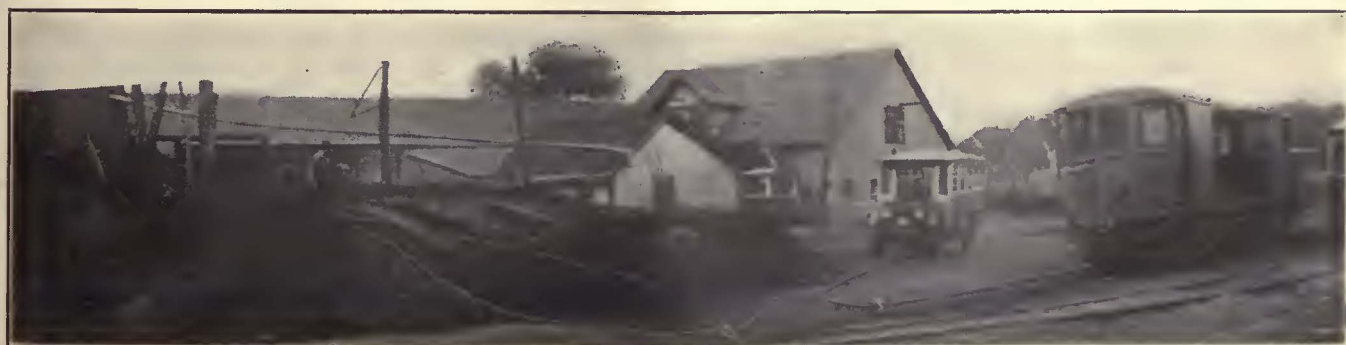
The Car Pulls the Shovel Loaded with Coal to the Top of the Pile and the Bus Pulls It Down
