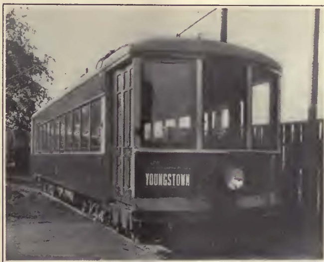
Both Entrance and Exit Are Normally by the Front Door, but an Emergency Door at the Rear Is Also Provided
