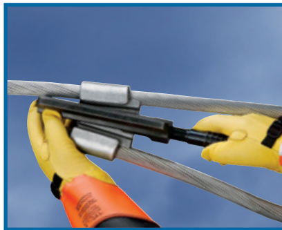
Place tool head assembly on connector and tighten.
