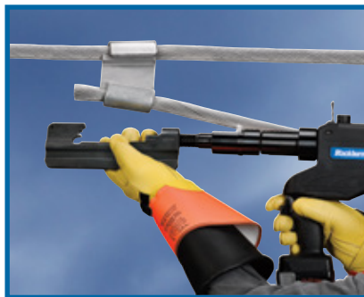
Release power unit trigger. Remove the entire tool assembly from the connection.
