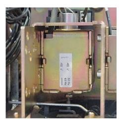
This is an electromechanical device that operates the operating mechanism's release lever after an electromagnet has energized, thus closing the circuit-breaker. When permanently powered, the shunt closing release accomplishes the anti-pumping function.
