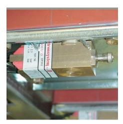
**First level - intervention for low pressure**: indication is given when the gas pressure drops from 380 kPa absolute to a value below 310 kPa absolute.
