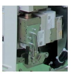
This is a mechanical device that allows the operation of the undervoltage release to be de-activated.
