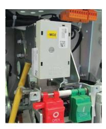
Similarly to shunt opening release -MBO1, this allows the opening command of the apparatus to be transmitted in the remote mode and can be energized by a circuit that is completely separate from release -MBO1.
