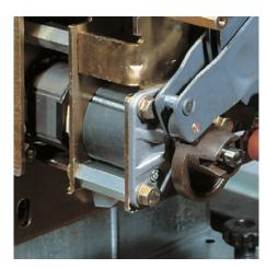
Automatically loads the springs of the operating mechanism after the closing operation.
