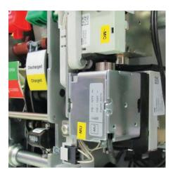
The undervoltage release opens the circuit-breaker when there is a sensitive reduction or lack of the voltage that powers it.
