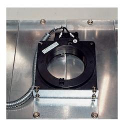
The external toroidal transformer is essential for detecting earth fault currents when the circuit-breaker is equipped with just two current sensors. It also allows earth fault currents of less than ten or so Amperes to be detected.
