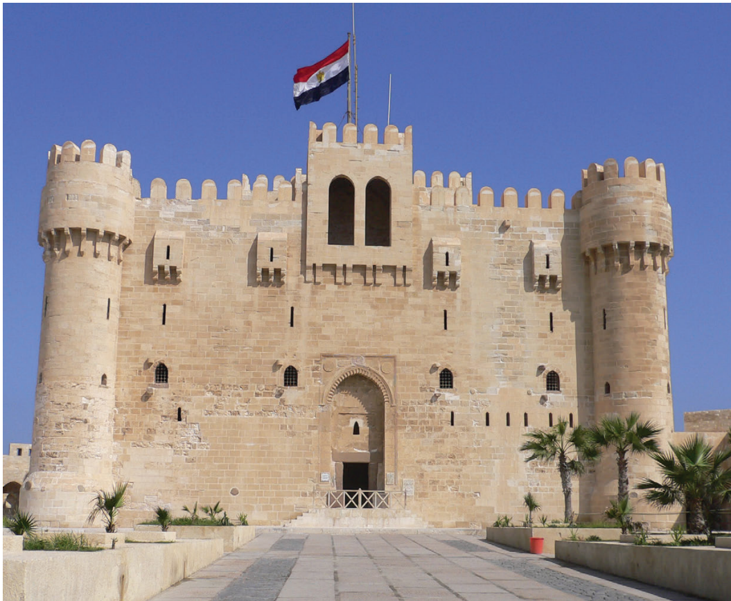
Figure 4: Photograph of the master tower of the citadel of Alexandria. (Photograph by the author.)
