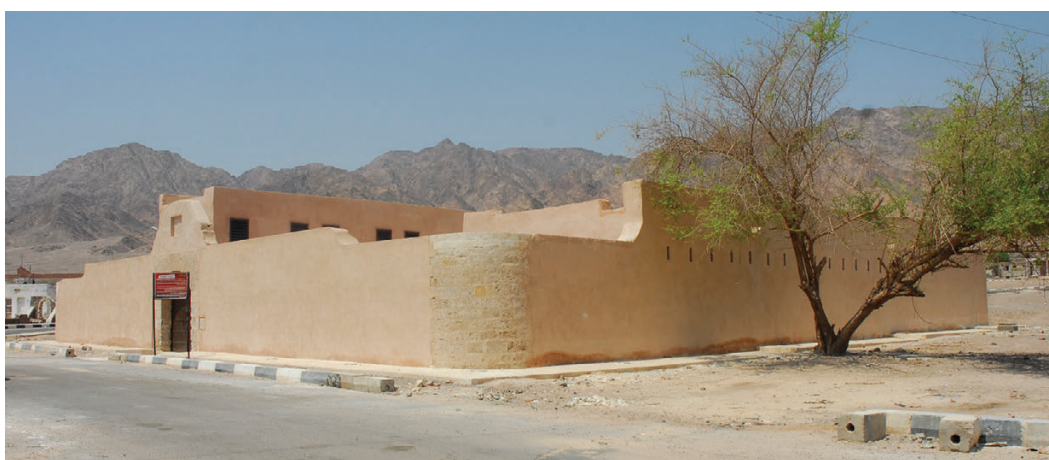
Figure 23: Photograph of the Nuweiba fort. (Photograph by the author.)
