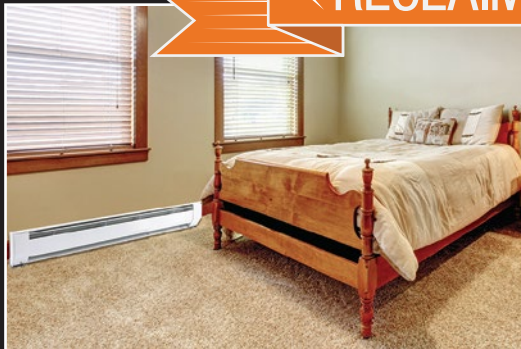
Standard Baseboard Heater
