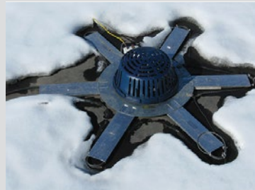
Roof/Drain De-icing System
