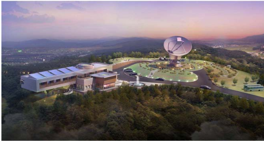
Figure 4. Bird's eye view of the KVG site.
