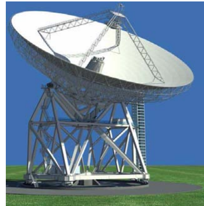
Figure 6. Artist's rendition of the structure of the Shanghai 65-meter antenna.
