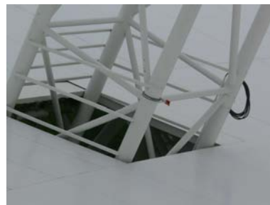
Figure 4. Retro-reflector on support leg.
