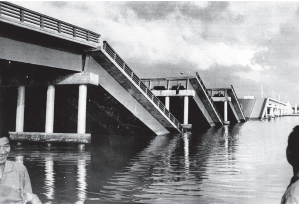
Figure 23.5 A bridge snapped into pieces after the magnitude-7.5 Niigata quake struck. Source: Keystone Pictures/ZUMA Press/Alamy.
