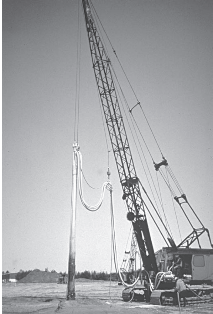
Figure 26.5 Crane lowering vibroflot into the ground (courtesy of Hayward Baker Inc.).
