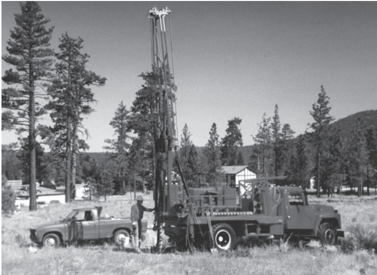
Figure 4.1 A truck-mounted drill rig.
