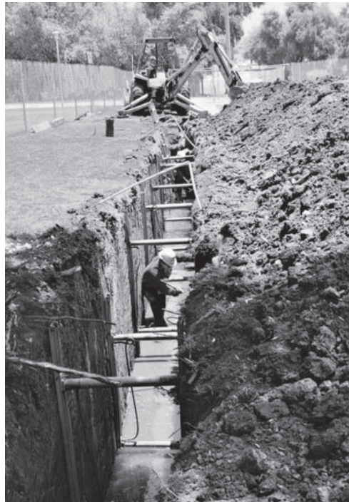
Figure 4.7 This exploratory trench was dug by the backhoe in the background, and has been stabilized using aluminum-hydraulic shoring. An engineering geologist is logging the soil conditions in one wall of the trench.
