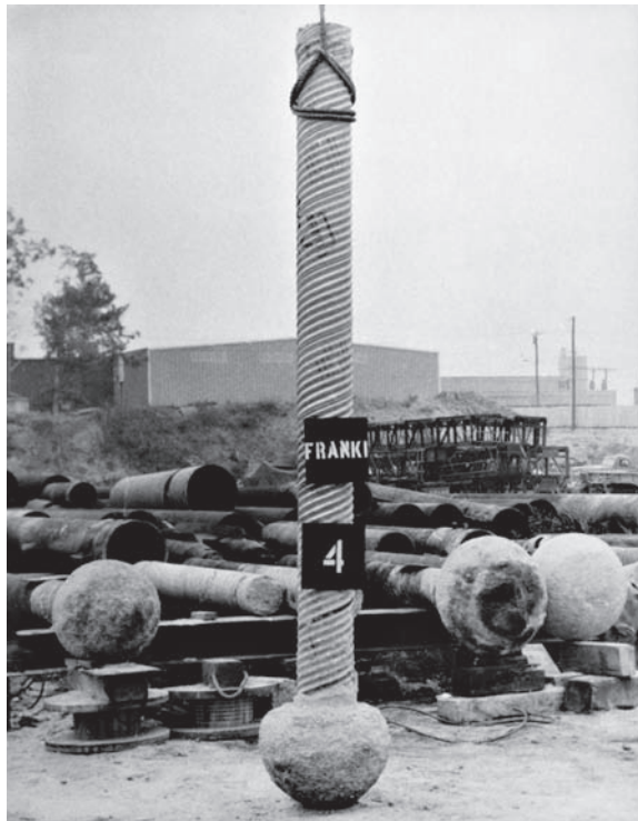
Figure 12.53 This “mini” PIF was extracted from the ground. It had a base diameter of 600 mm (24 in) (photo courtesy of William J. Neely).
