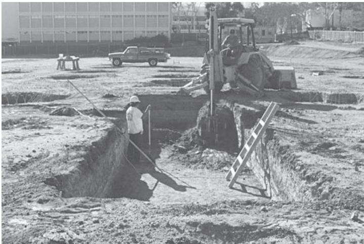
Figure 6.7 A backhoe making an excavation for a spread footing.
