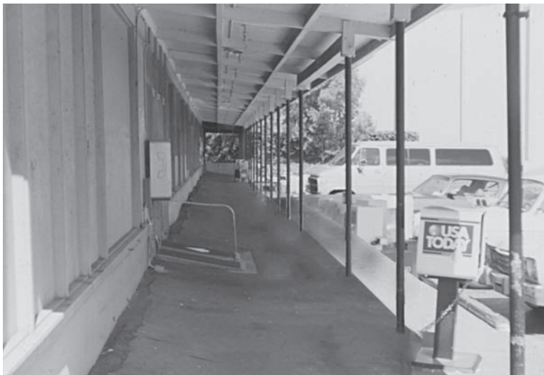
Figure 23.4 The ground around this pile-supported supermarket settled about 400 mm in twenty five years, but the building remained at essentially the same elevation. This required continual maintenance around the perimeter of the building. Note the steep slope to reach the front door and the spacer blocks required at the top of the footing supported posts which settled with the surrounding ground.
