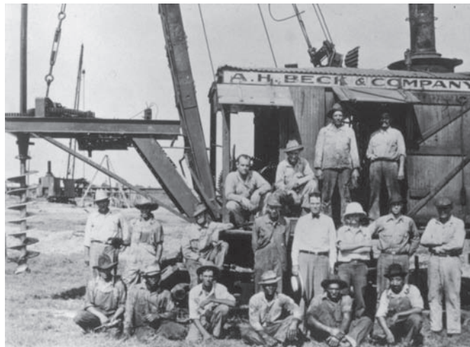
Figure 12.28 Early truck-mounted drill rig and crew, circa 1925 (ADSC: The International Association of Foundation Drilling).
