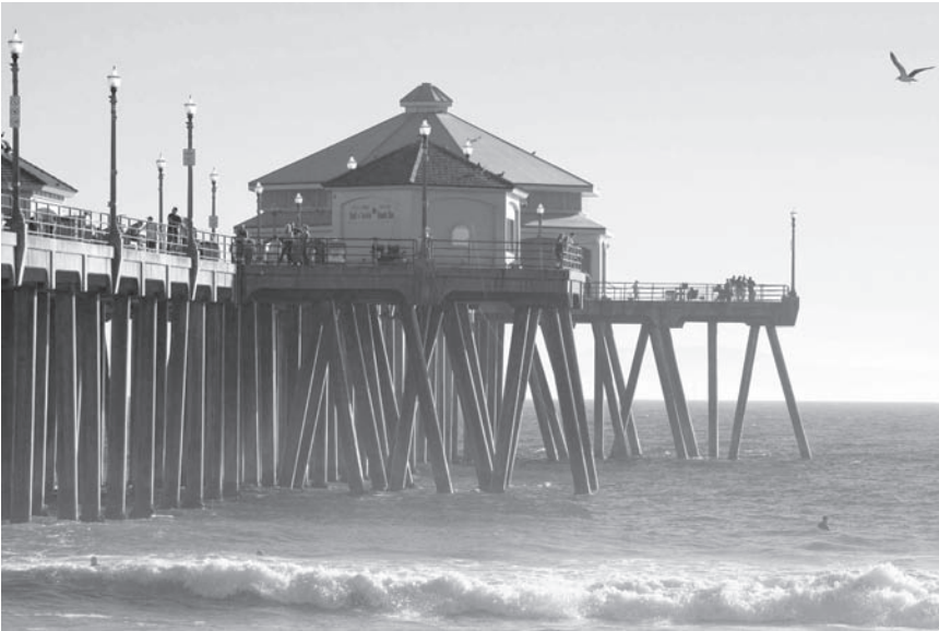
Figure 22.2 Prestressed concrete battered piles at Huntington Beach pier, California.
