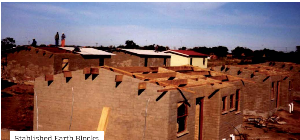
Stablished Earth Blocks
