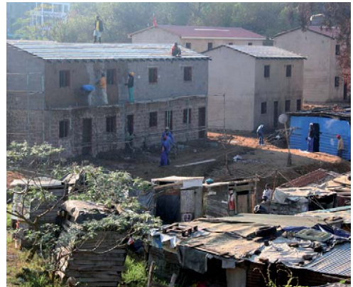
A typical informal settlement upgrading process utilizing a double storey attached low cost typology and a 'rollover' upgrading approach (i.e. site developed in small 'rollover' phases to minimize temporary relocations requirements) (Cato Crest).
