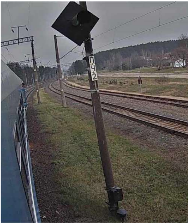
Fig. 1. Marking plate of the railway traffic light
