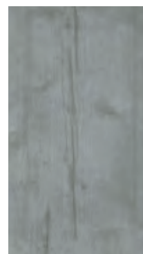
Concrete Door Finish
