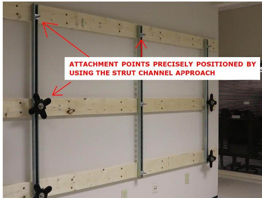
Figure 6 – Wall mounting installation with Strut channel profiles.
