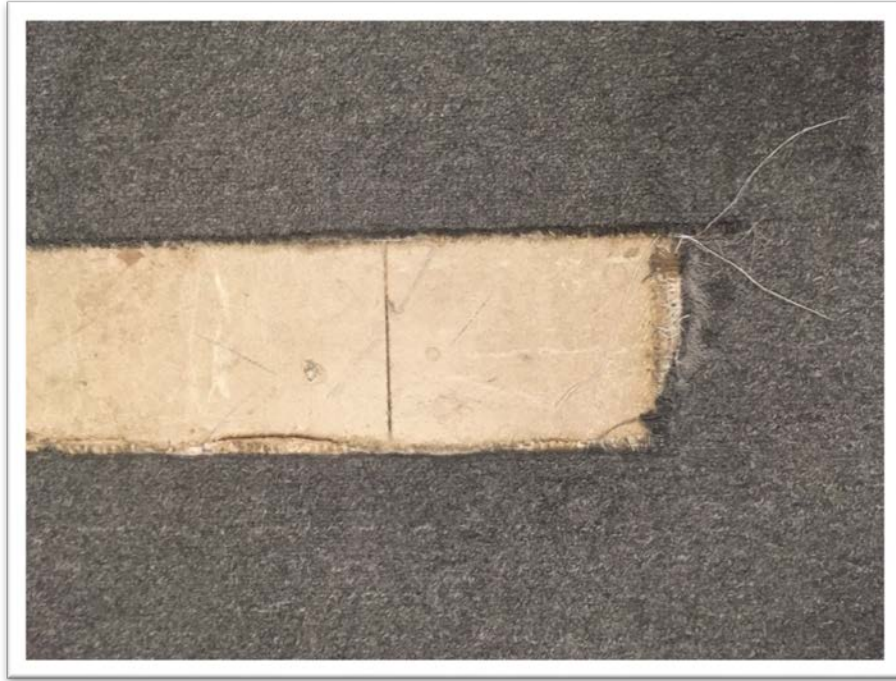
9 x 9 Floor Tile/Black Mastic under Carpet in Rooms 3, 4, 5, 6, 8, 9/Unknown Quantity
