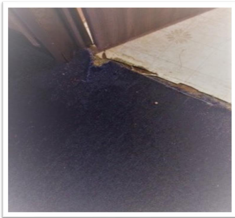
White and Beige Vinyl Flooring with Mastic in Latrine and Room 5
