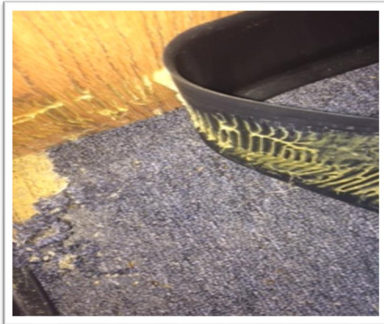
Black Cove Base with Mastic throughout the building lower walls
