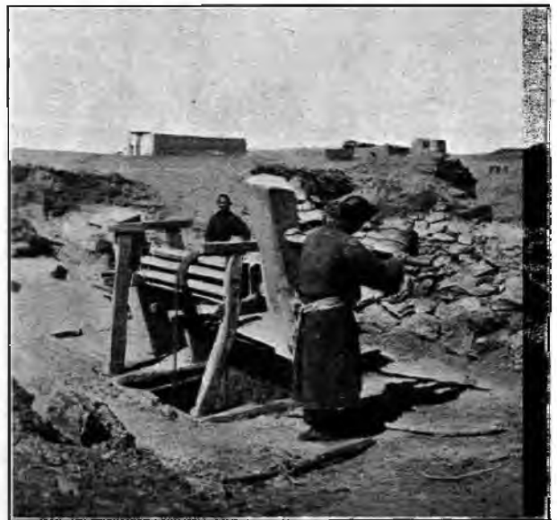
Coal Mines at Shih-kou-i. The shaft is 150 feet deep. Man power alone is used.
