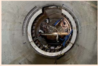
Figure 4. Compartment plug under installation during the MPT.
