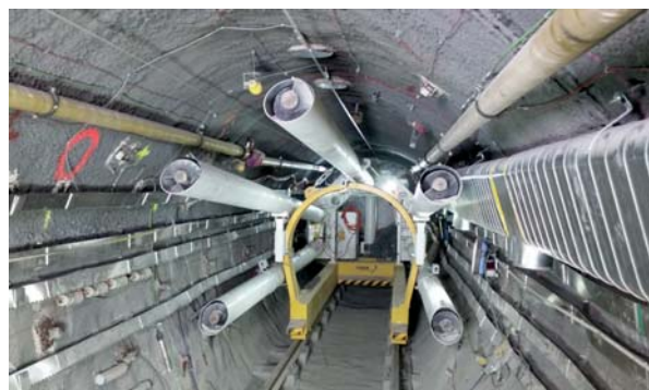
Figure 5: Backfilling machine front in the FE emplacement tunnel
