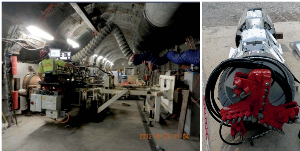
Figure 3. Excavation of the cell (left) using the auger drilling machine (right).
