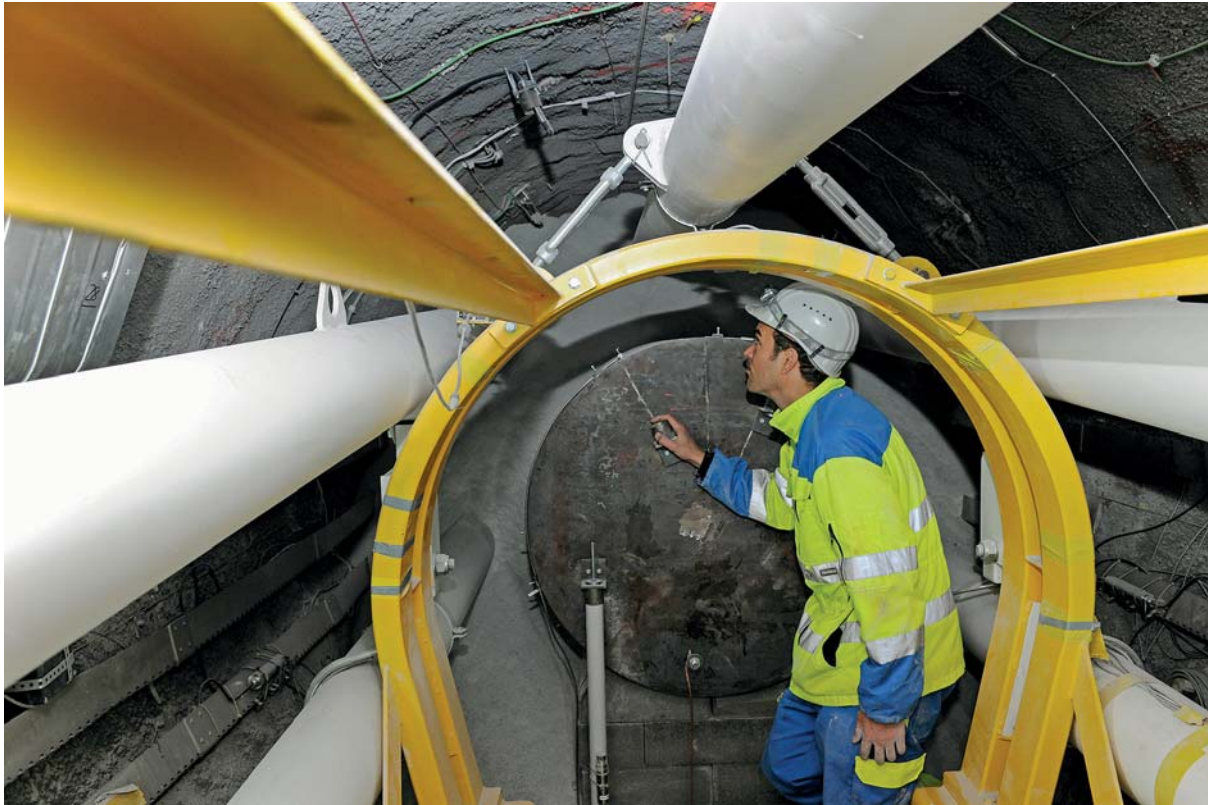
Figure 8. Photo of granular bentonite emplacement at Mont Terri rock laboratory. Steel canister (Heater), emplacement machine (5 augers), granular bentonite, Tobias Vogt (Nagra).
