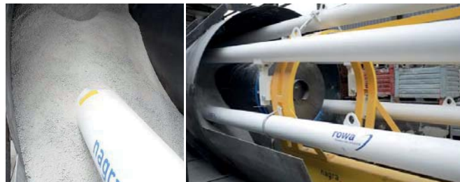
Figure 4: The newly developed backfilling machine being tested in a 1:1-scale tunnel model in an off-site workshop. The 1 m diameter dummy heater can be seen in between the augers.
