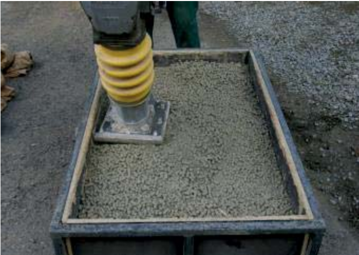
Figure 6. Compaction testing with a vibrating tamper.
