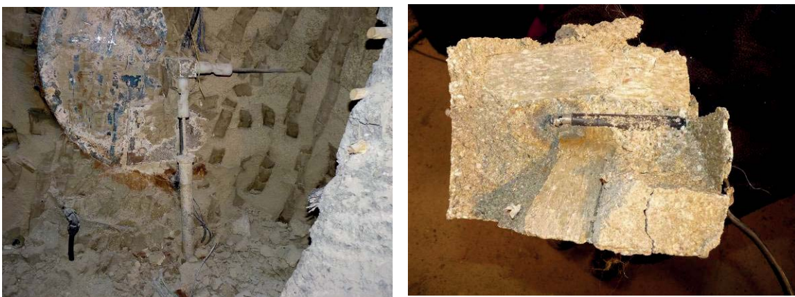
Figure 2. Sensors appearance during the dismantling of the EB experiment at Mont Terri (extensometers on the left hand side and water content sensors on the right).
