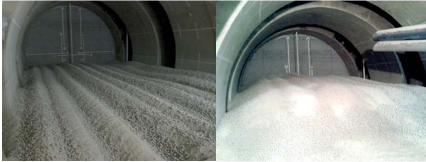
Figure 7 The swelling clay core emplacement operations
