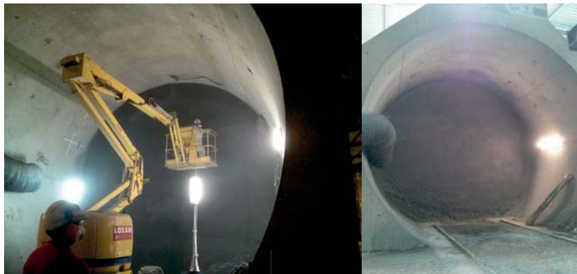
Figure 8 The low pH shotcrete containment wall construction (spraying/ left; end product/right)
