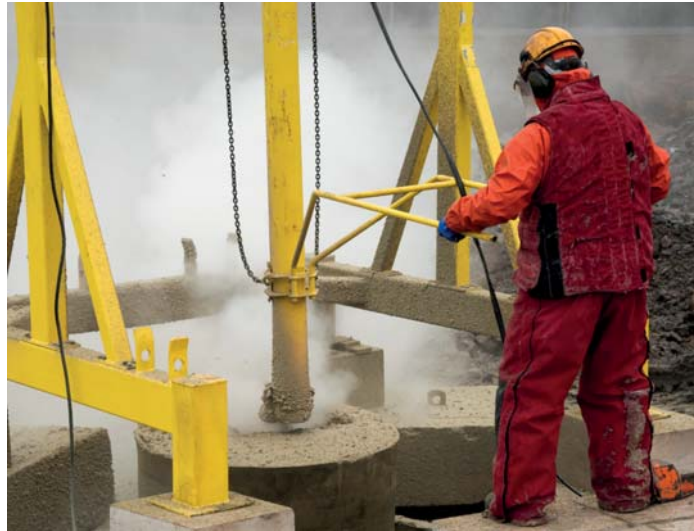
Figure 4. Testing of bentonite block water-jet cutting method.
