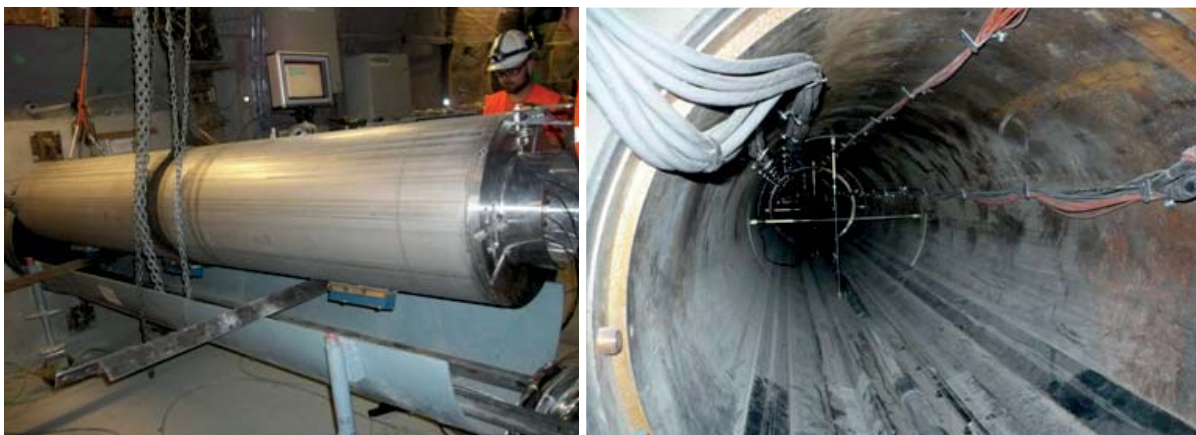
Figure 4. Heater installation (left), instrumented sleeve (right).
