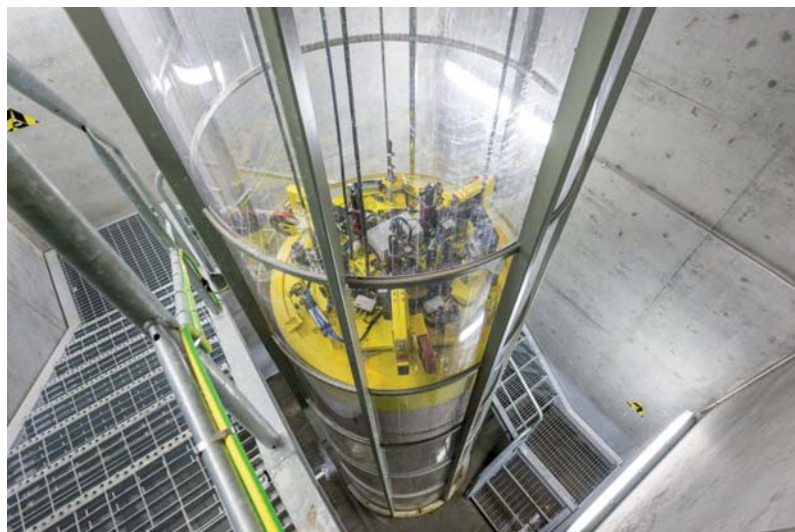
Figure 5. Installation of concrete block to full scale disposal hole in test hall, which is located in ONKALO area.
