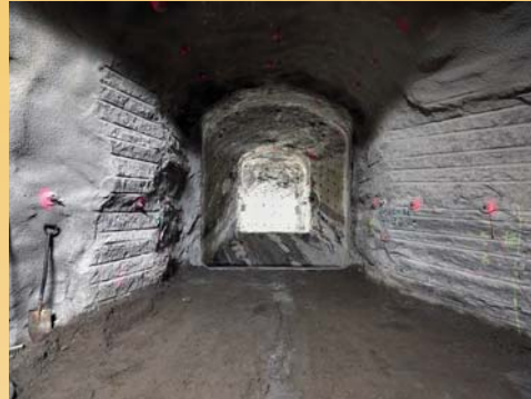
POPLU Experiment plug location is ready for installing and casting activities. © Posiva
