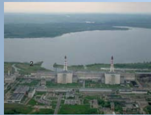
Ignalina nuclear power plant
