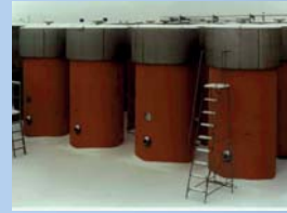
Existing SNF storage facility
