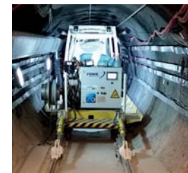
Figure 8: Breaks attached to the rails
