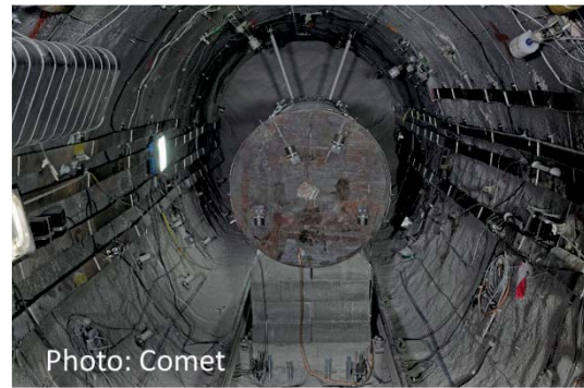
Figure 8: Emplaced bentonite blocks in the FE tunnel: bentonite block wall in the interjacent sealing section and bentonite block pedestal sustaining a heater.
