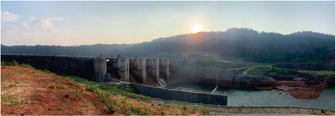
Photo 2.1. The Dam for the Nam Theun 2 Hydropower Project
