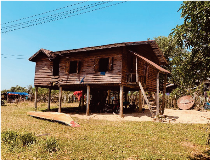
Photo 2.4. A Typical Resettled Dwelling in the Nakai Plateau
