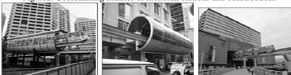
Figure2. Coordinating manner of monorail stations and constructions
