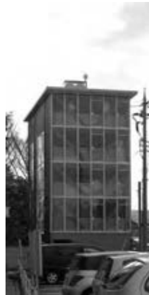
Photo.1: External view of Kanazawa M Bldg.
