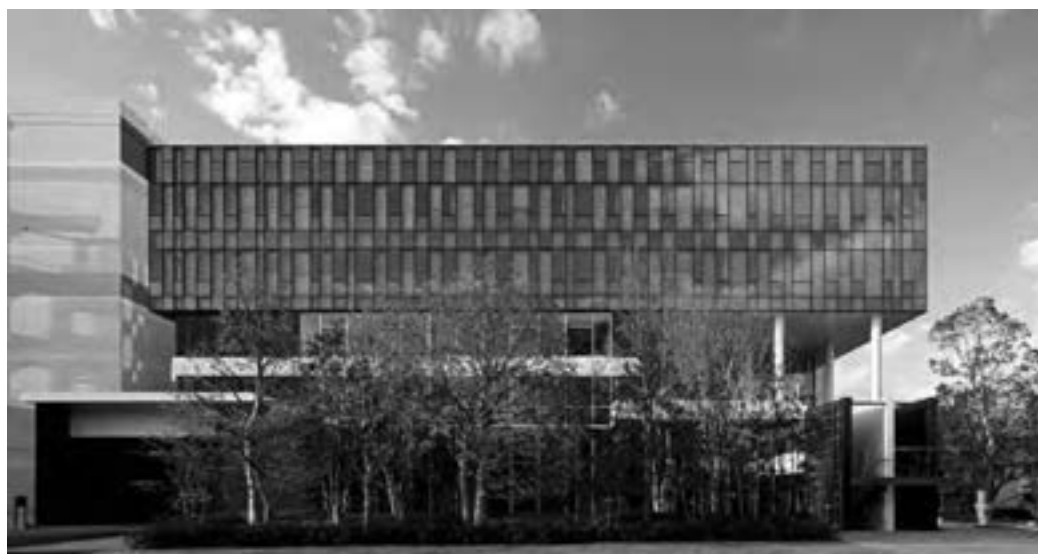
Photo 3 : “Kasukabe Convention Hall” Bldg. (Photo by YAMASHITA SEKKEI INC.)
