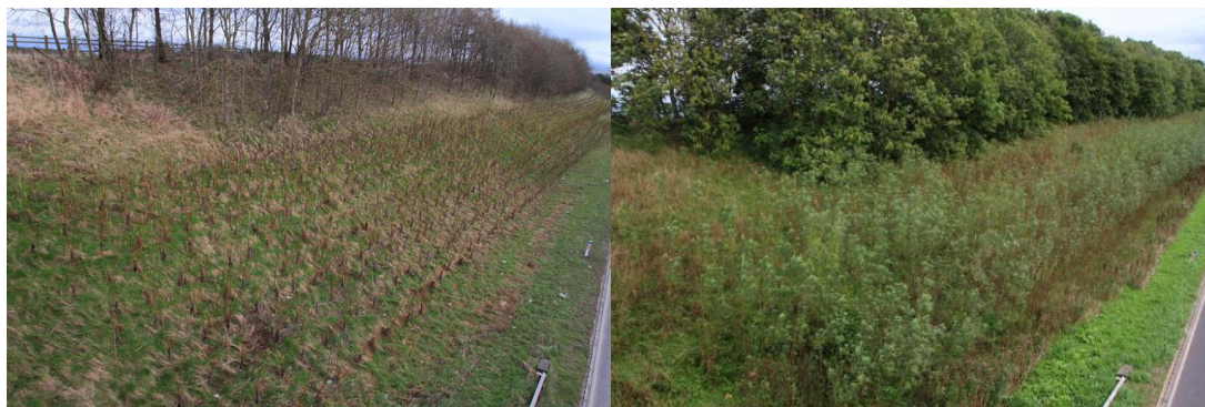
Figure 1. General view of the M6 south of J40 from the B5320 overbridge looking south-east: Left, March 2017 (installation was between November 2105 and February 2016); Right, August 2018 showing growth.
