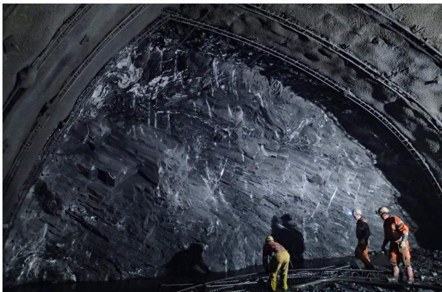
Figure 1: Calcareous Schists from Bündner Schist Unit used for aggregate production during tunnel driving;
