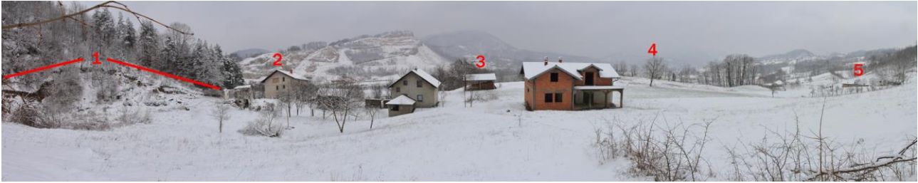
Figure 2. Panoramic image showing (1) the northerly lateral margin scarps (red lines indicate the clearest scarp features do not reflect the full complexity of the landslide) with (2) significantly damaged buildings, (3) buildings with relatively less damage in the central portion of the landslide, (4) tree demonstrating the lifting of the frontal lobe, (5) at the extreme right the roofs of buildings at the southern lateral margin of the landslides are evident.
