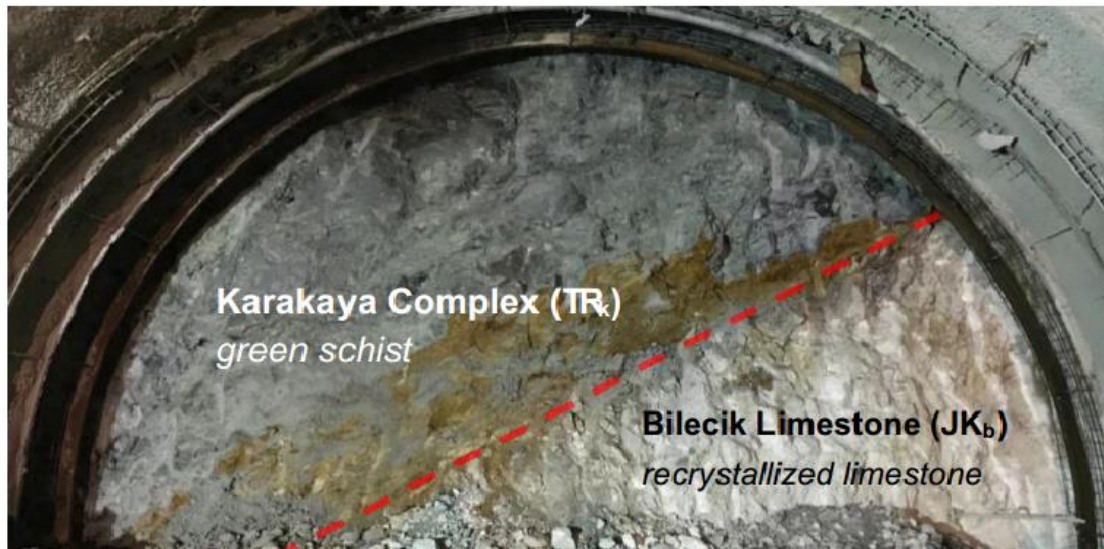
Figure 1. Appearance of tectonic boundary between the geological units at the tunnel face
