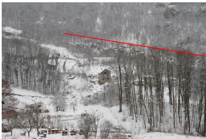
Figure 1. Scarp features at the northern lateral margin of the landslide (the red line indicates the most evident parts of the scarp features but is not intended to reflect the full complexity of the landslide). Damaged buildings are also evident.
