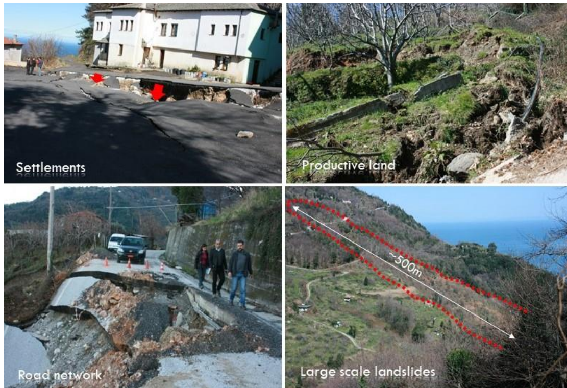
Figure 1. Typical aspects of landslide damage within northeastern Pelion area
