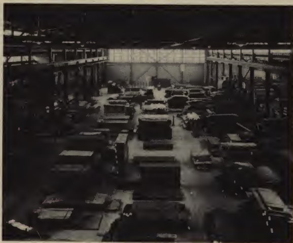
Looking down the oversize center bay from the catwalk of Fullerton's 80-foot overhead crane. This crane is equipped with an electronic scale which automatically weight-stamps each load. Ample floor spaces allow fast, efficient movement of stock to shears or shipping dock.
