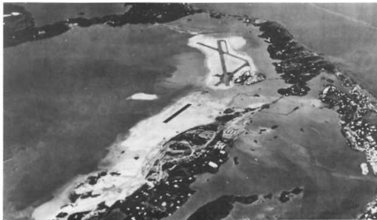
Kindley Field, built primarily on dredge fill in Castle Harbor adjacent to Long Bird Island, Bermuda, as it appeared in April 1942.
