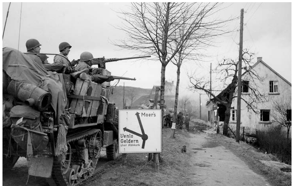
Vehicles of the 5th Armored Division, Ninth U.S. Army, pass a crossroads sign in Vord, Germany, with burning buildings in the background, 3 March 1945.
