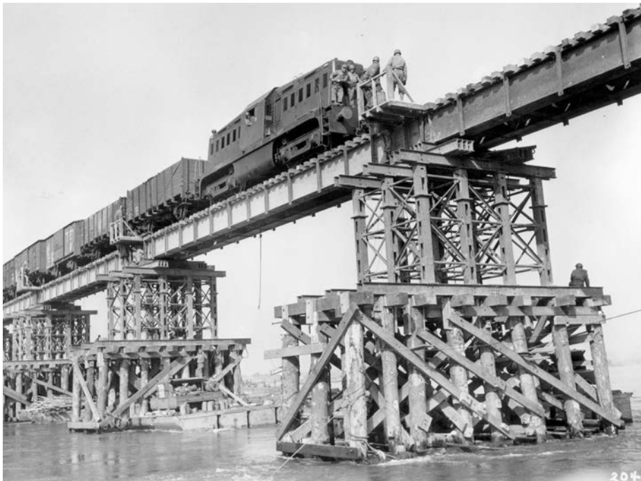
A Transportation Corps train crosses the Rhine River on a new bridge at Wesel.
