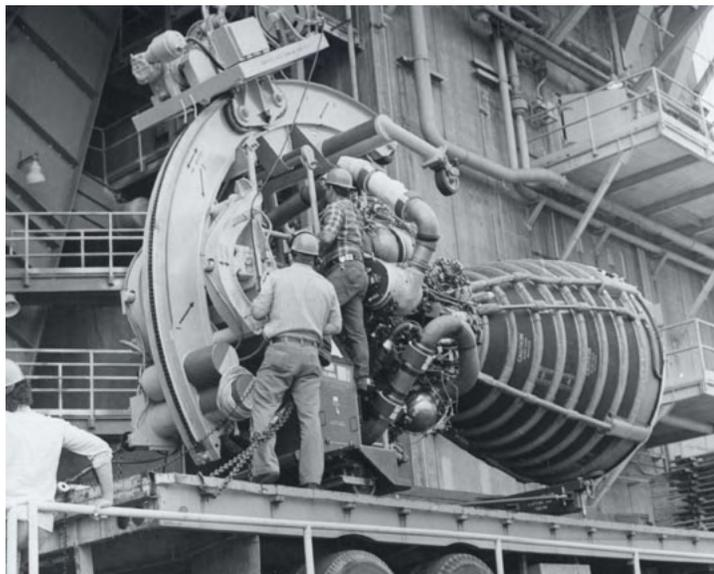
**Photo 2.2.** SSME hoisted into the A-2 test stand at Stennis Space Center (then, NSTL) before undergoing test firing, January 1, 1979.
