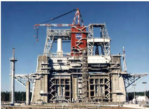
B-1 (left) and B-2 (right) Positions Configured for SSME Testing.
