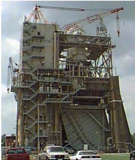
A-1 Test Stand Configured for SSME Testing.
