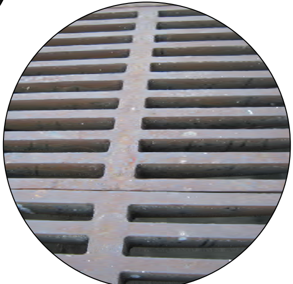
Figure 3-30: Typical Original Grating
