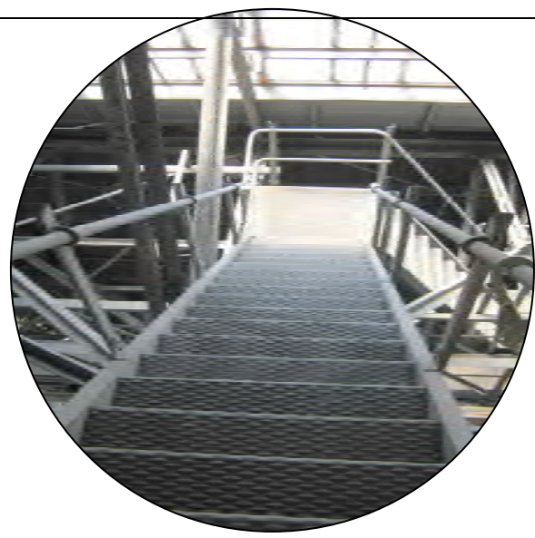
Figure 3-2: Stairs Between Catwalks
