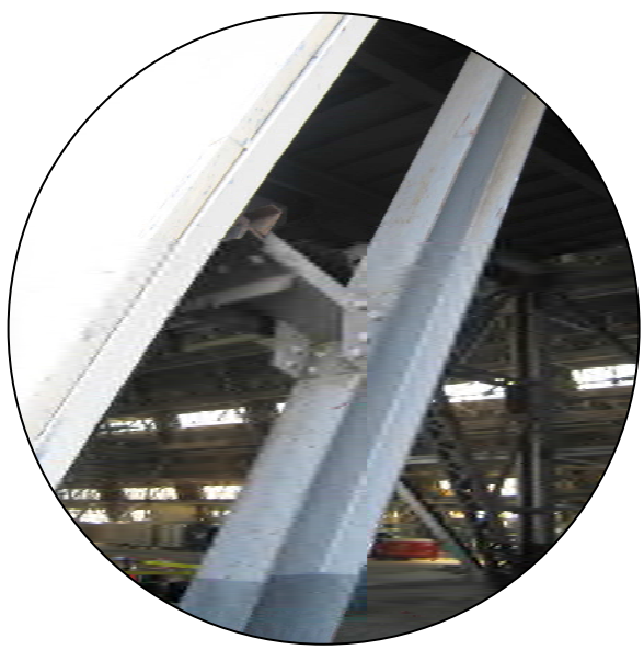
Figure 3-4: Wind Girt @ 7'-6" O.C.
