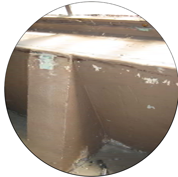
Figure 3-16: Concrete Wall at Hangar Perimeter, From Inside
