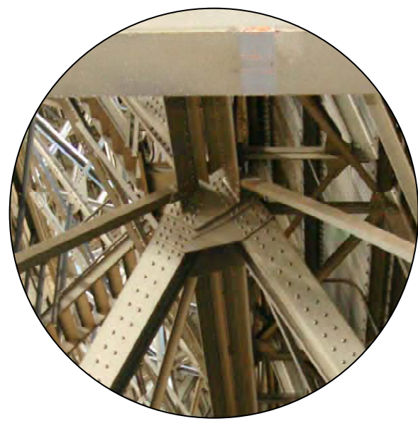
Figure 3-6: "A" Frame Top Connection
