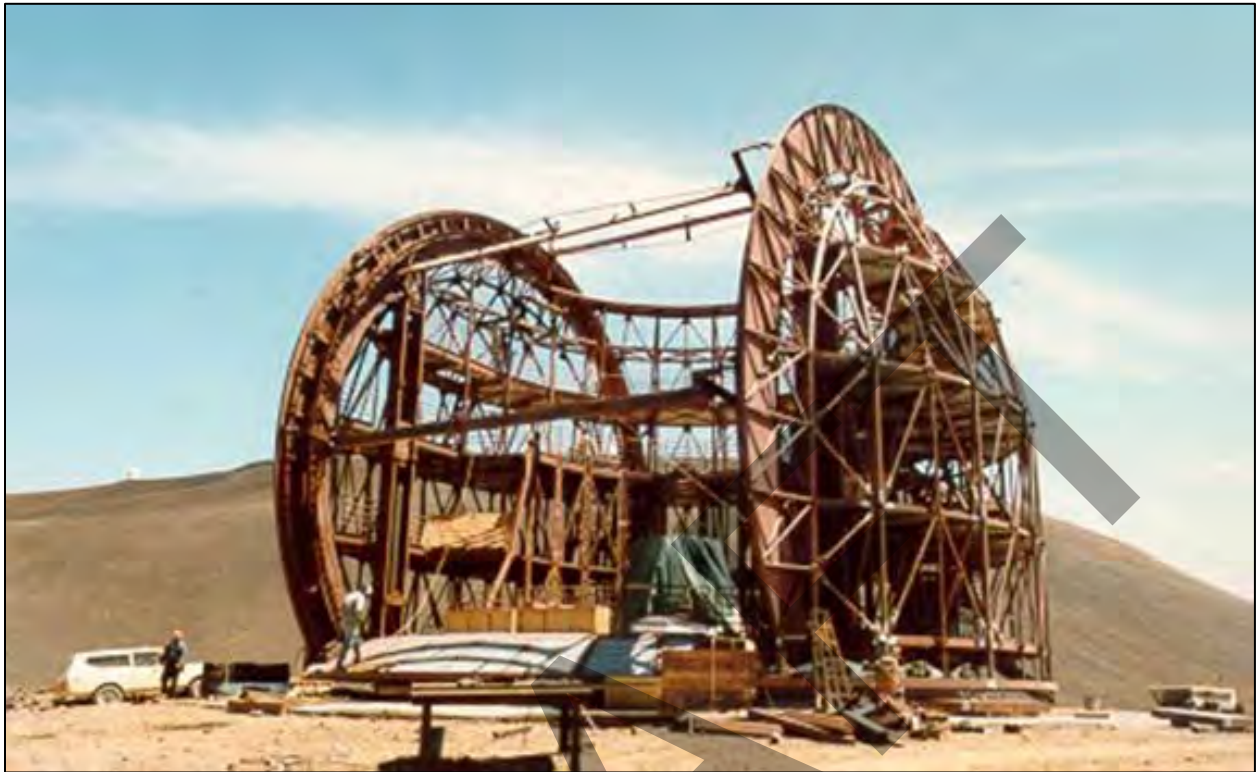
Figure 5-5: CSO's Internal Structure During Construction
