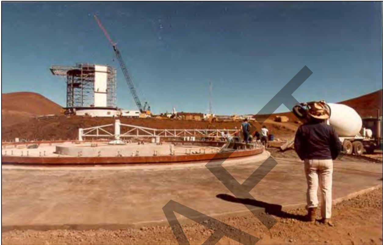
Figure 5-6: Photograph of CSO's Foundation During Construction
