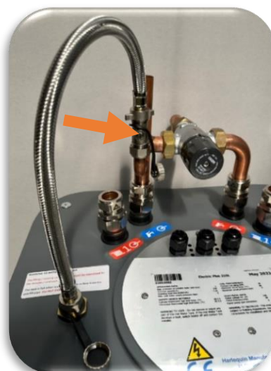
Figure 5 Filling loop connected
