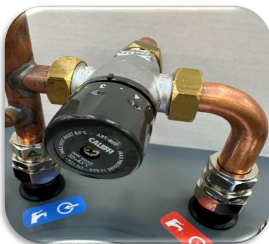
Figure 2 Thermostatic mixing valve settings
