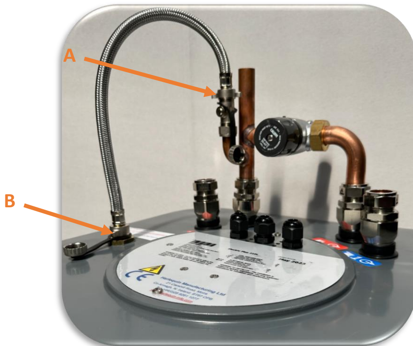
Figure 14 Hot and cold-water connections
