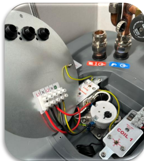
Figure 16 Control compartment layout
