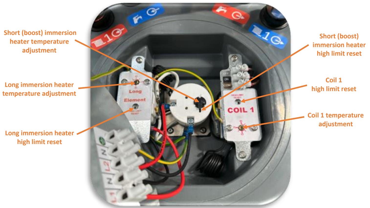
Figure 4 Location of thermostat controls
