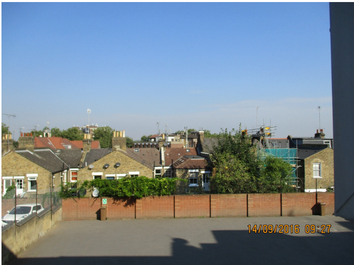
View of properties to rear (north) of site, illustrating fall in land levels.
