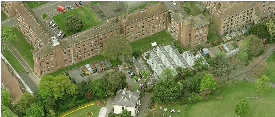
Fig 2: aerial view of existing buildings and greenhouse
