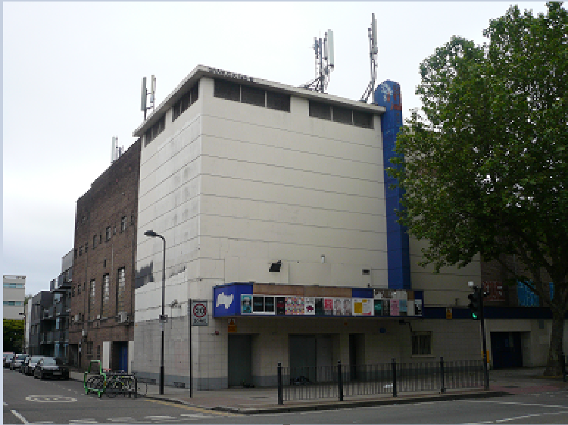
Front elevation – looking east
