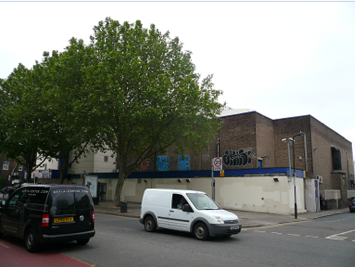
Front elevation – looking west
