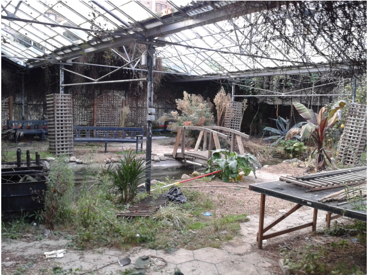
Fig 4: internal view of the existing greenhouse
