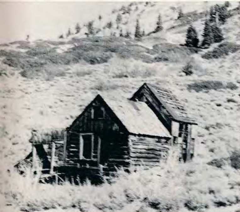
Remains of the "Half House" Saloon where the $10,000 bill was used as "credit" and pasted on the wall by Matt and "Butch." This presented an accounting challenge that eventually forced the owner out of the saloon business. Money came from Nat'l. Bank of Denver.
