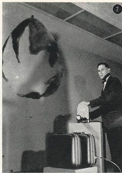
Ray gun fits in suitcase, yet one pulse of Laser light of 1/2000th second duration cut through steel plate to burst balloon 10' beyond. It may also burst balloons of bombast and threats frequently launched from behind Iron Curtain.
