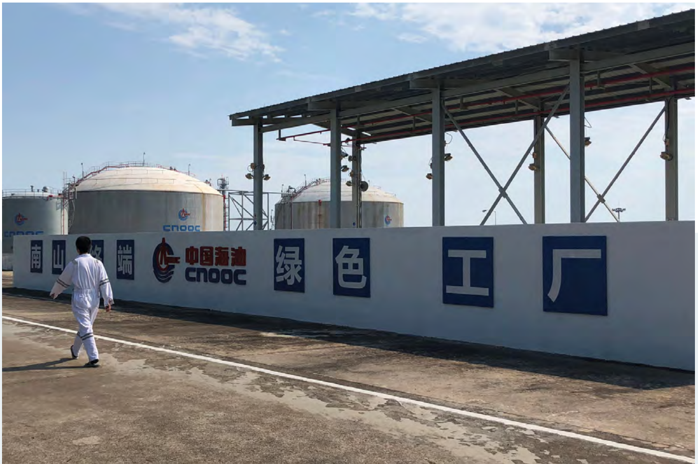
Nanshan LNG terminal in Hainan. Image: Muyu Xu / Reuters.
