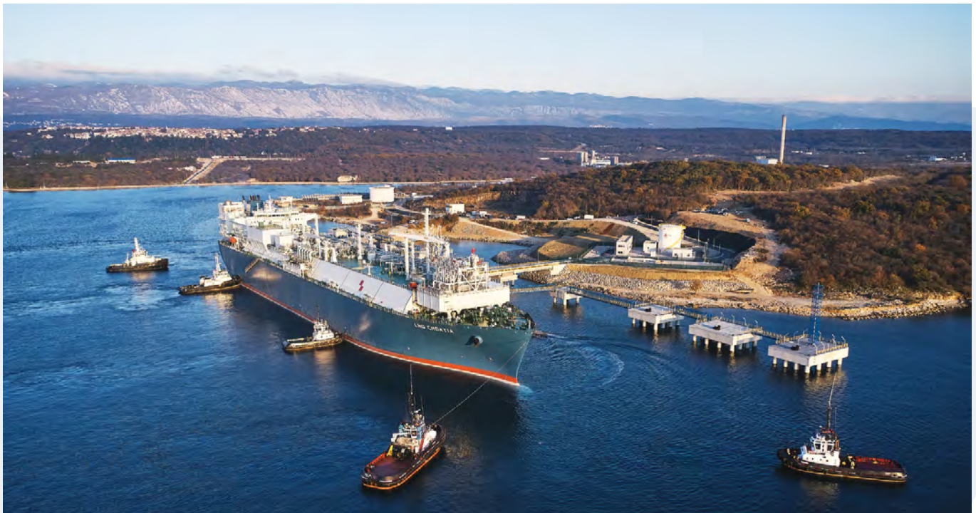
Croatia's first LNG terminal is located in Omišalj, on the island of Krk in Croatia. Photo courtesy of LNG Croatia LLC.
