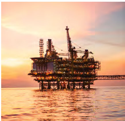
Figure 1. The Central Processing Platform takes production from four wellhead platforms and routes it to the Terengganu Gas Terminal plant onshore. Image: Hess Corporation.
