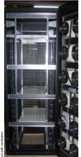
Reck with ventilation
