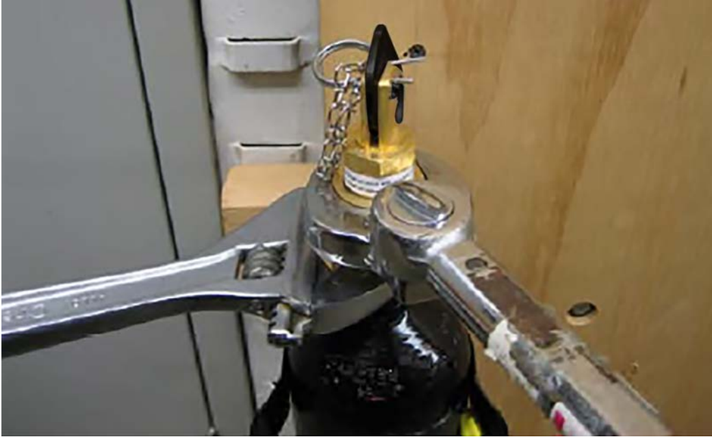
Figure 2. Lever Operated Head (P/N: WK-870652-000) tightened using Torque Wrench with 1-1/2” Crowfoot. Always use black lever style per Bulletin 16-24K.
